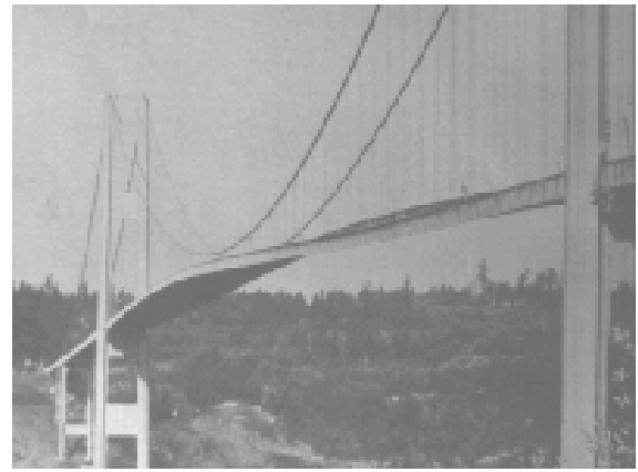
Figure 1, An Example of Resonance, The Tacoma Narrows Bridge Collapse
